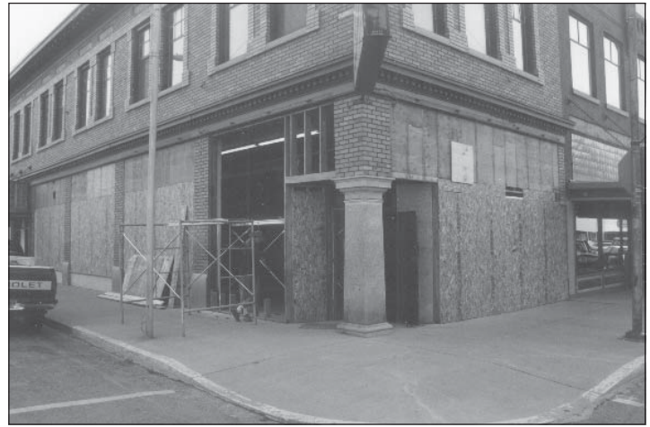
Boarded up after dryvit removal.
