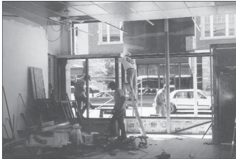
Constructing the recessed doorway.
