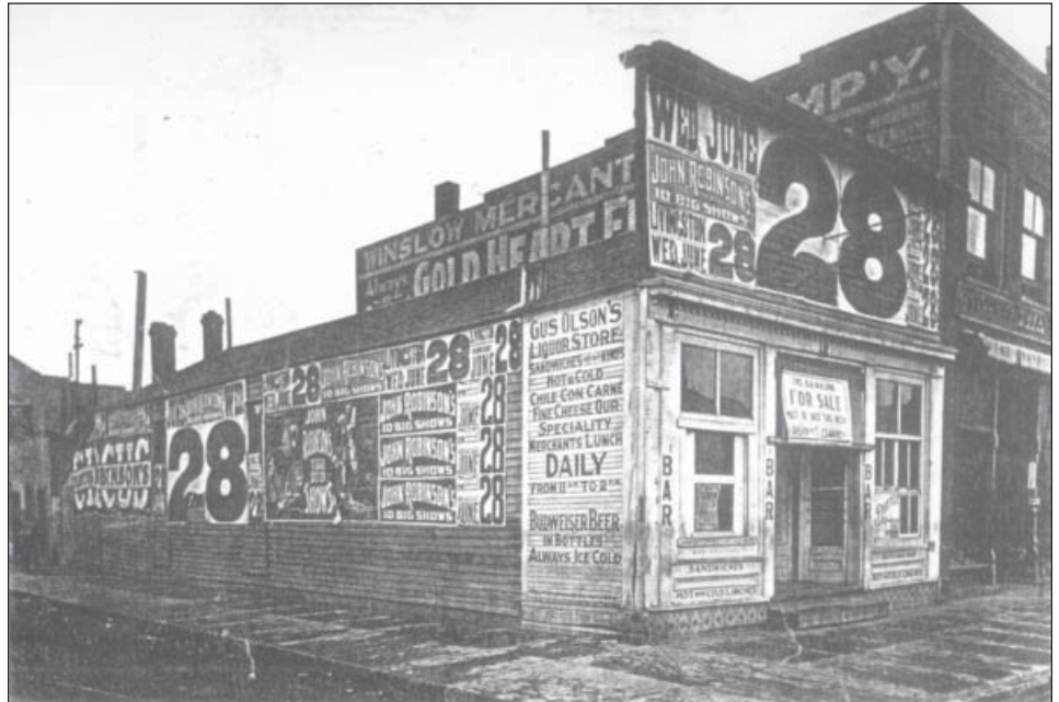
A REALLY bad example of signage! Shortly hereafter the Historic Preservation Committee closed this business for bad taste and flagrant violation of preservation rules and regulations. (Original building at 101 south Main-A bar and Cafe owned by Gus Olson: Demolished June 21, 1916.)
